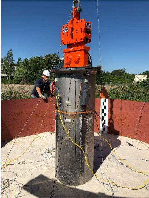
Fig. 2: pile extraction with APE Model 3
