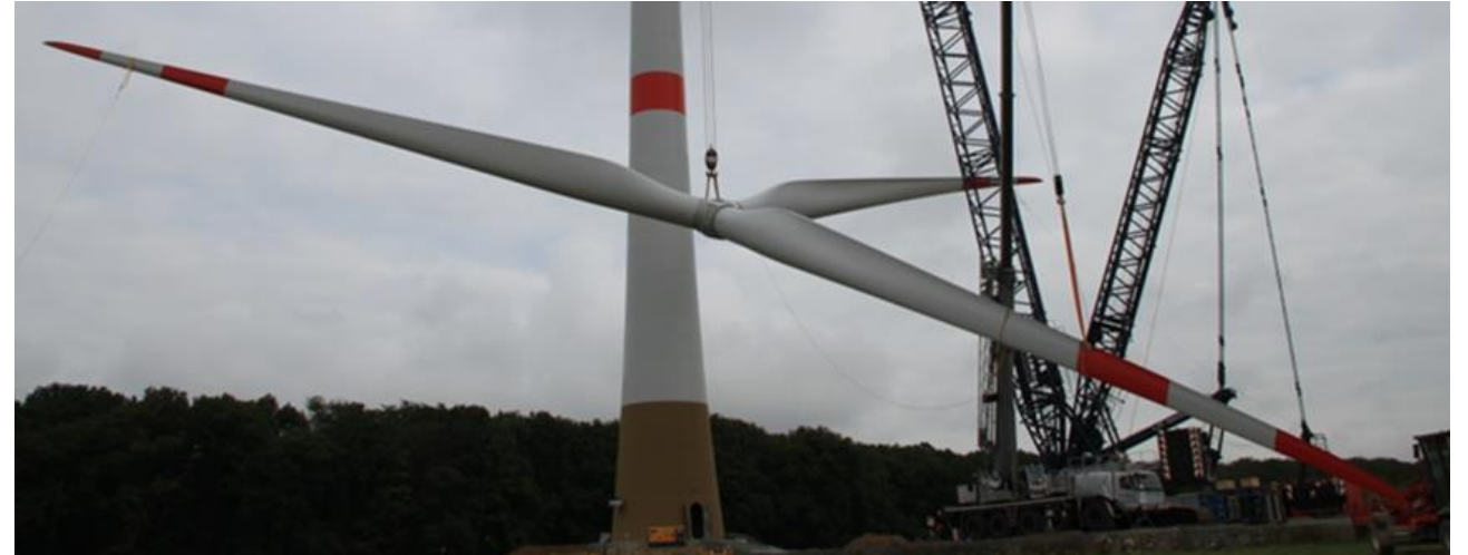
Pick-up of the rotor of a wind turbine with 117 m diameter
