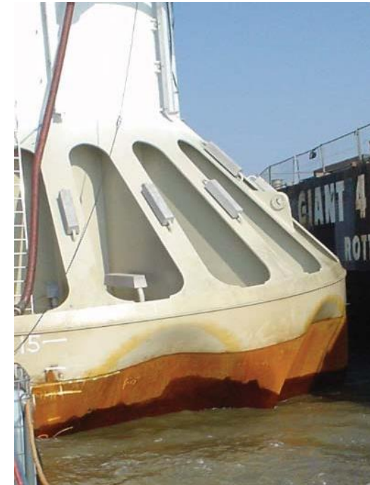
Buckling failure (Monopod)
